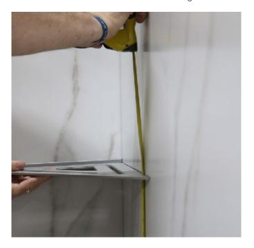
Using a level, mark location where corner shelf is to be installed on the Nuance panels. (Recommend the Corner Shelf would be installed 43" from the shower floor).
