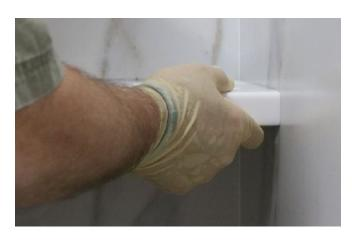
Avoid large gaps between the Nuance surface and corner shelf by sanding. or cutting to ensure good fit to wall panels. Apply wooden support blocks (4) with hot melt to under location where corner shelf is to be mounted.
