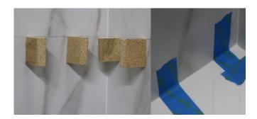
Place a piece of blue painters tape on top of support block, so that sealant does not prevent removal of support blocks after cured.
