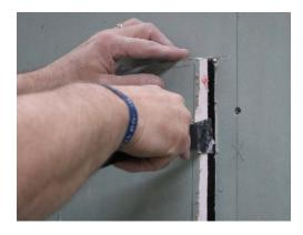
Cut and remove the current substrate (tile, green board, cement board) to expose the wall structural framing. Cutout should be no larger than 1/4" larger than the dimensions of the recessed niche.
