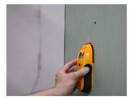
Determine location of recessed niche (Standard height for the recessed shelf would be 43" from the shower floor to the bottom of the opening).
